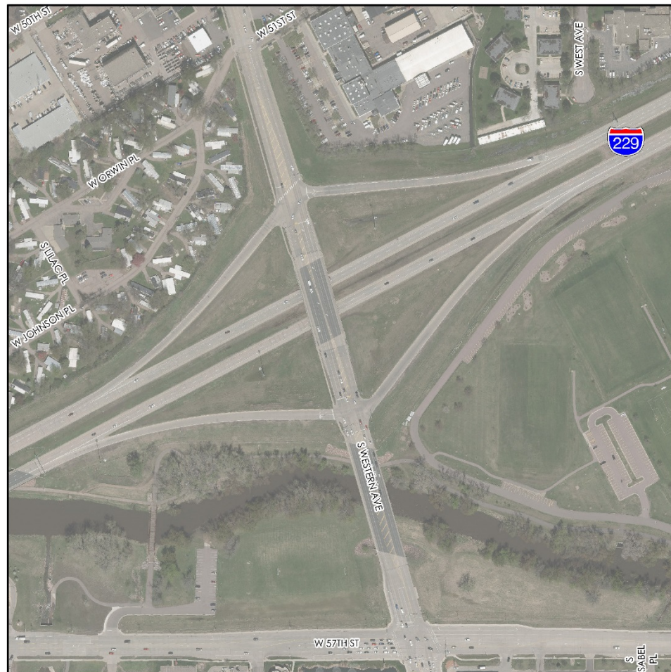
Figure 6 – Existing I-229 at Western Avenue Interchange
